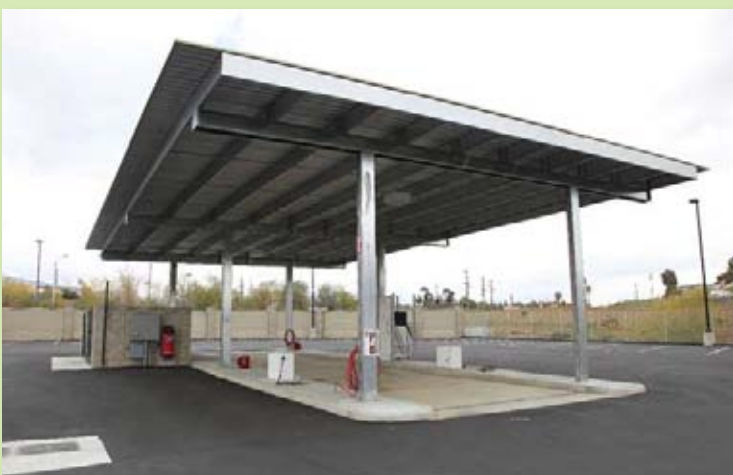
The wash bay area also includes a solar canopy.
