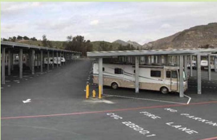
The facility features 144,000 square feet of solar canopy atop 400 storage units.
